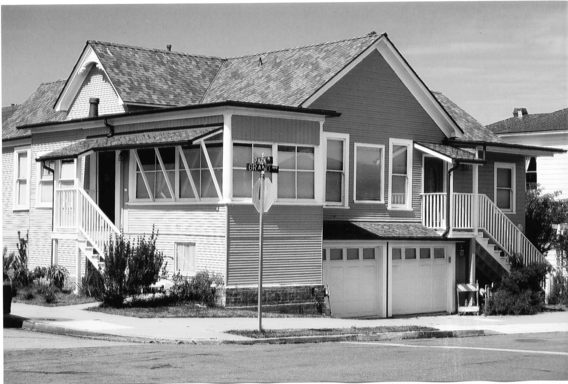
Photo #1. Looking NW at the south facing facade & east side-elevation, note modern porch additions, staircases, window additions & double garage doors below grade, Kent Seavey, September, 2019.
