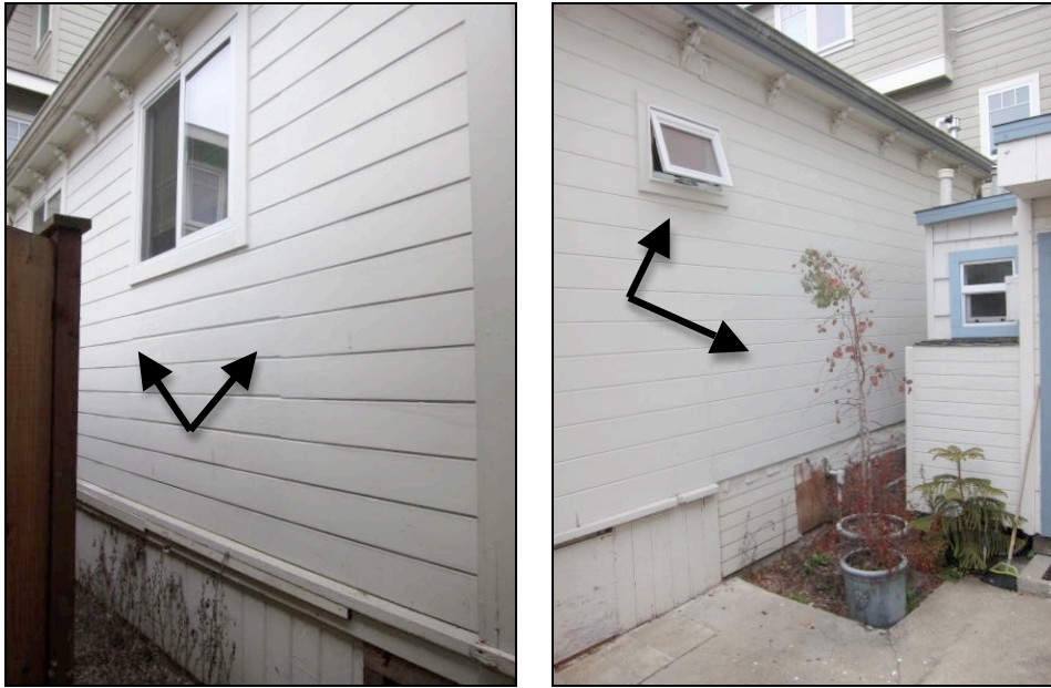
Figures 10 and 11. Left image details the north elevation's circa-1905 rear addition, showing the replaced wood siding installed when the window openings were modified (arrows). Right image details the south elevation at the guesthouse, showing replaced siding boards and a new window opening (arrows).
