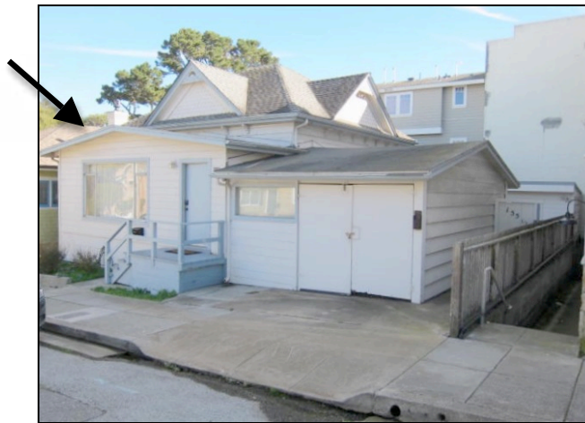
Figure 12. View of front elevation showing locations of proposed changes. The garage will be removed and replaced with a parking structure. The 1958 porch addition (arrow) will be remodeled and a new front entrance and entry porch constructed. The gable roof will be converted to a shed roof in order to see the existing Victorian cornice brackets.
