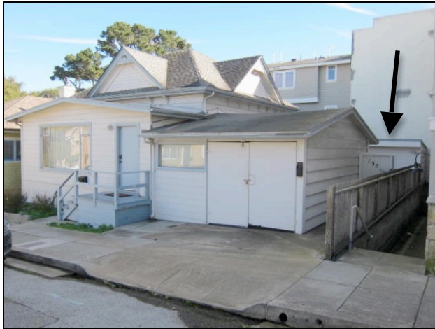
Figures 6 and 7. Left image shows the front (west) elevation with circa-1958 gable-roofed and garage additions dominating the front elevation. The guesthouse is located behind the garage (arrow). Right image details the north elevation, showing an original window surround and one-over-one, double-hung sash (arrow).
